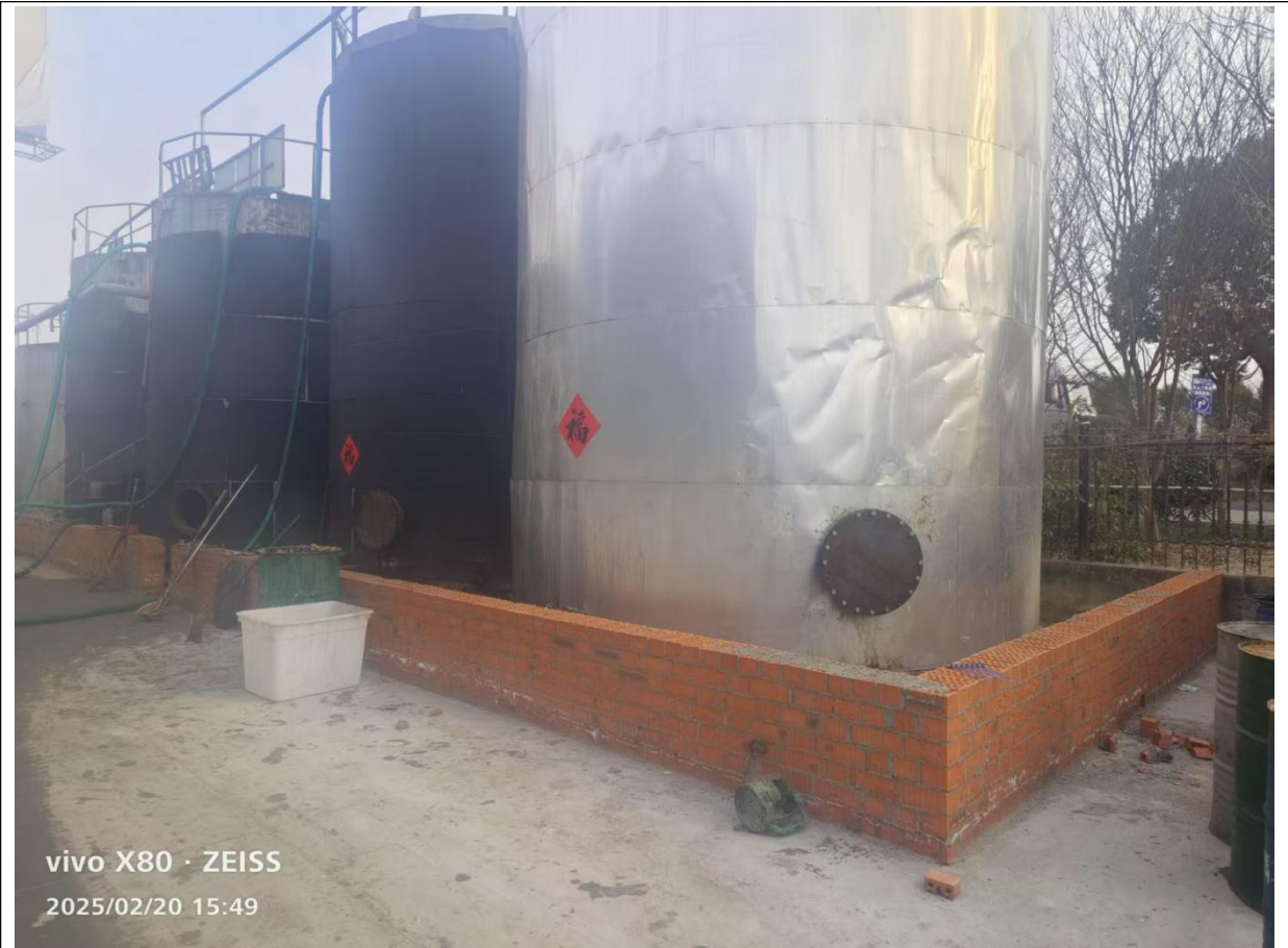
油脂儲罐圍堰
